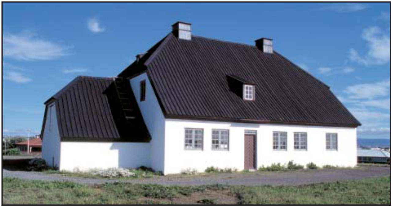
Nesstofa by Seltjörn pond, near Reykjavík, built of stone in 1761-1763. The residence of the first Surgeon General of Iceland and also housed the first authorized pharmacist in Iceland. The architect of the house was the Danish court stonemason, Jacob Fortling. Acquired by the National Museum in 1979.
