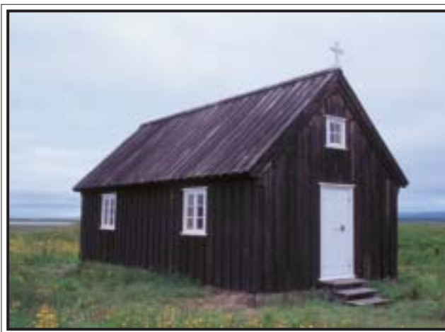
Sjárvarborg Church in Skagafjörður, north Iceland. It is of the older type of churches without a tower, built in 1853. Acquired by the National Museum in 1972.
