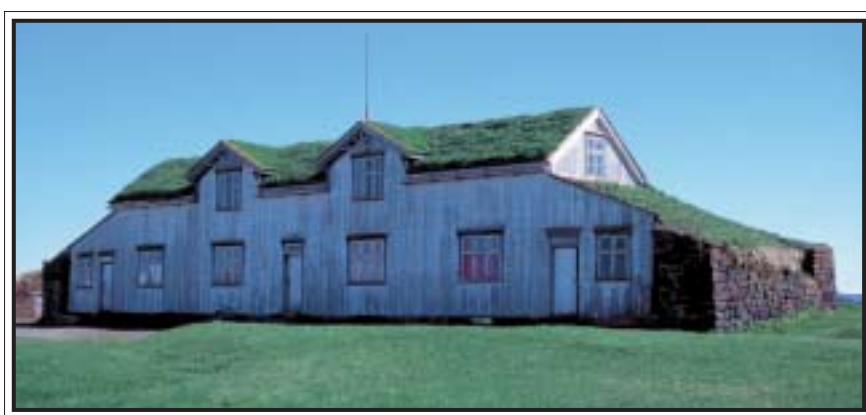
Grænavatn in the Mývatn area, north Iceland. An impressive facade constructed about 1913 for a turf house, of which only the walls now remain. The house was built for two families, and shows the influence of the rural style of the area. Acquired by the National Museum in 2000.
