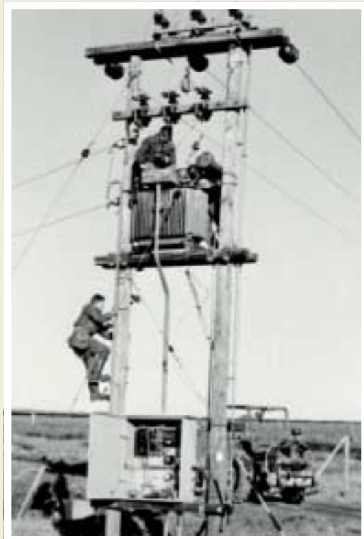
A big boost to northwest Iceland! Increasing voltage from 11 to 19 thousand volts in 1971.
