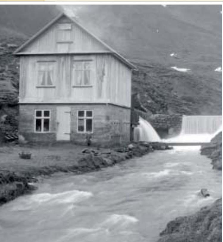
Hydropower station at Vík, southern Iceland, 1914.
