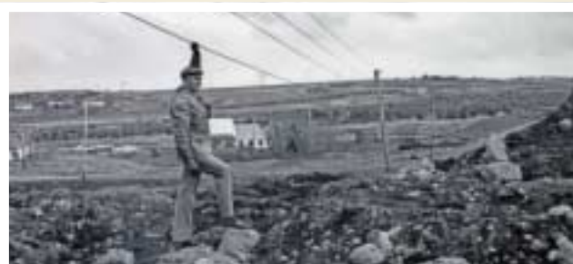
Do not try this at home! Checking the wires on the outskirts of Reykjavik in 1977.
