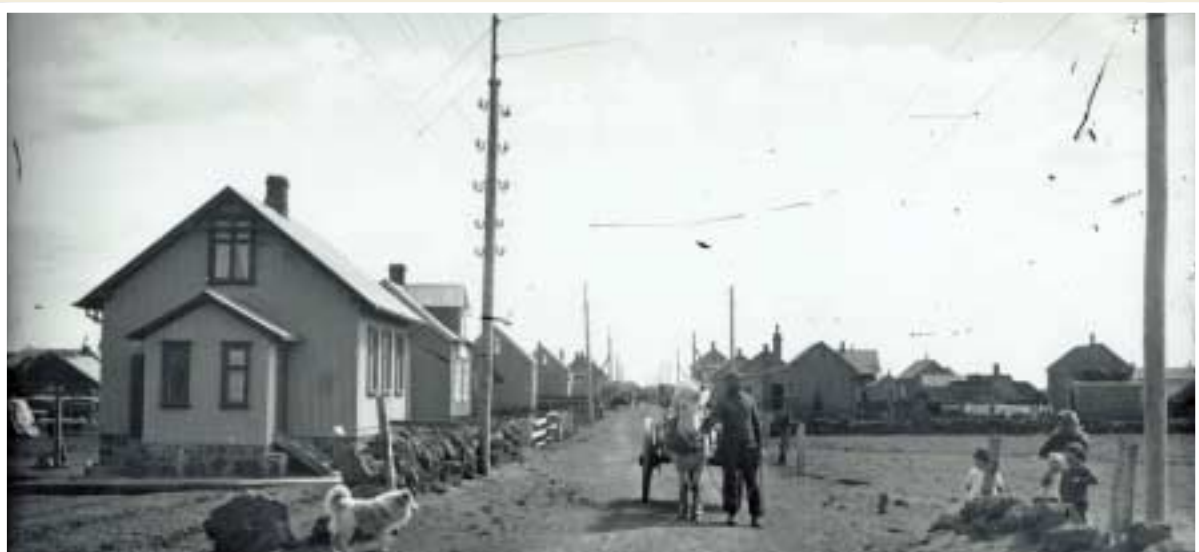
Early integration of power and telecommunications. Powerlines on extensions to telephone poles at Eyrbakki in south Iceland 1920.
