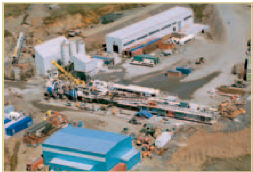
TBM ready for action outside Adit 2
