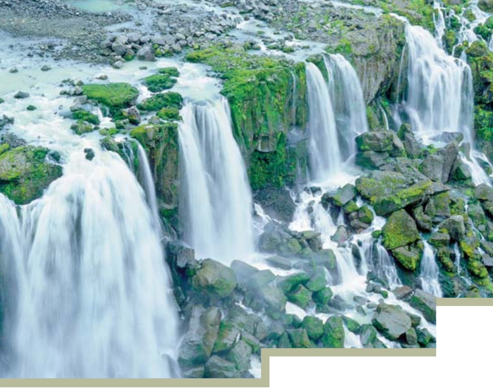
Groundwater springs forth in the Sigalda canyon below Krókslón reservoir. Unexpected man-made beauty!
