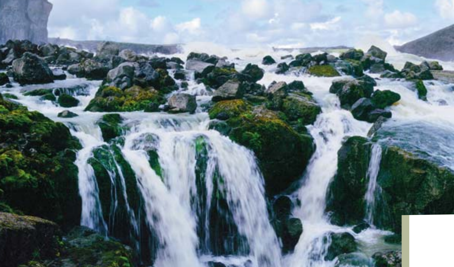
When reservoirs are filled beyond capacity, the water runs off through a spillway. This results in a diversity of waterfalls, as demonstrated by the man-made scenario of these falls below Krókslón reservoir, belonging to the Sigalda station.
