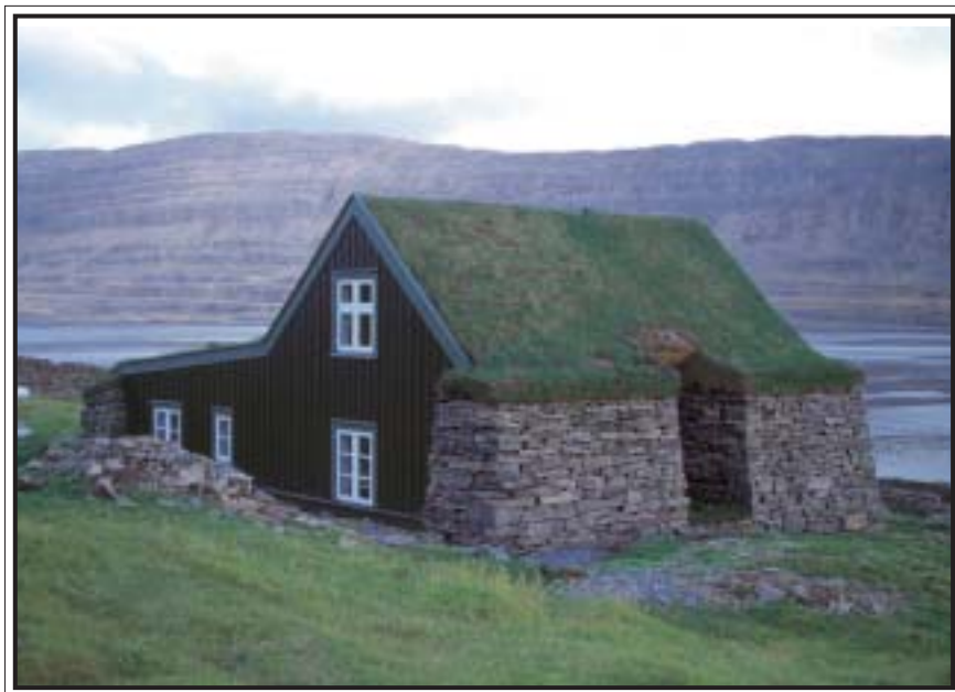
Litlibær cottage in Skötufjörður, north-west Iceland. A wooden house built in 1896 with stone walls on the long sides and a turf and grass-covered roof. Originally two families lived in the house, which therefore had a wall inside to divide it down the middle. Acquired by the National Museum in 1999.
