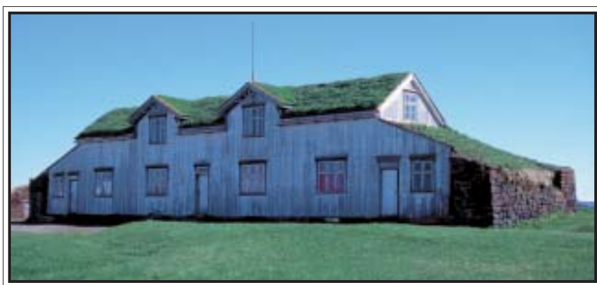
Grænavatn in the Mývatn area, north Iceland. An impressive facade constructed about 1913 for a turf house, of which only the walls now remain. The house was built for two families, and shows the influence of the rural style of the area. Acquired by the National Museum in 2000.
