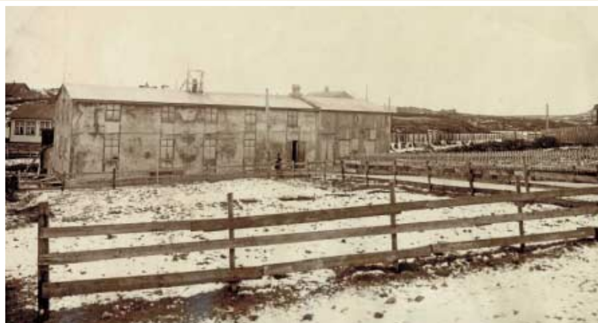
Unlikely beginnings! Jóhannes Reykdal's carpenter's shop housing the first hydrostation in Iceland in 1904. He sold electricity to nearby houses. There were no meters so he rented out the light bulbs.
