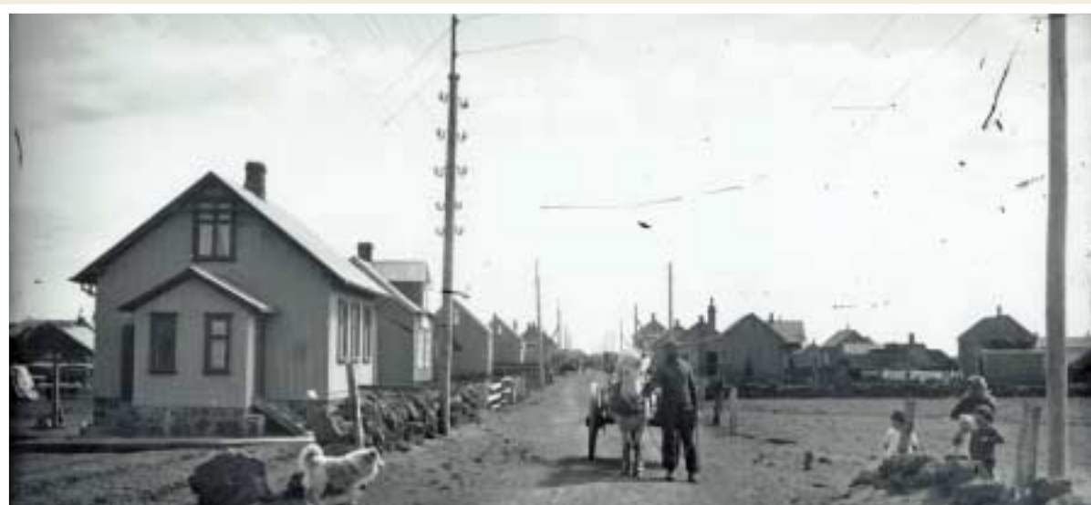
Early integration of power and telecommunications. Powerlines on extensions to telephone poles at Eyrbakki in south Iceland 1920.
