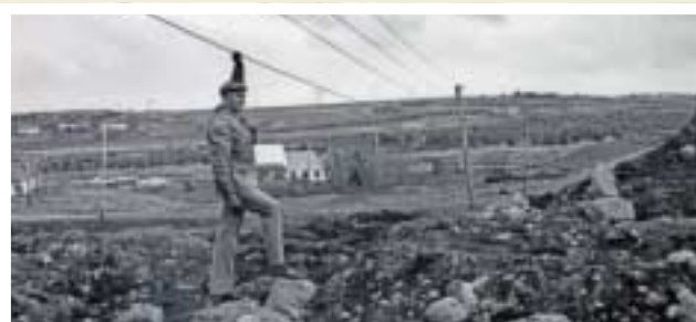
Do not try this at home! Checking the wires on the outskirts of Reykjavik in 1977.
