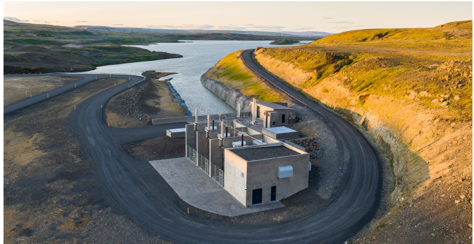
↑ Búrfell Station II Landsvirkjun's newest power station, Búrfell Power Station II, started operations in 2018.
