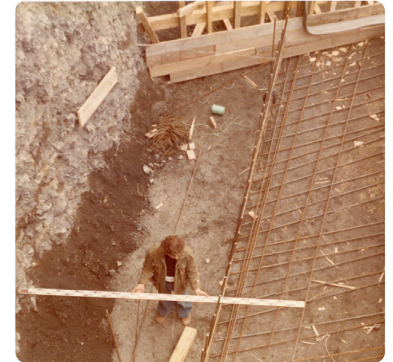
Construction at Sigalda in July 1976.
