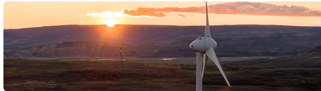
We have operated wind turbines at Hafíð, above Búrfell, since 2013, and experience shows strong performance in the area. Photo: Garðar Ólafsson.
