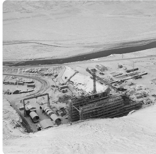
Búrfell Power Station under construction in 1967. Picture: Ólafur K. Magnússon.
