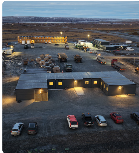
Ten foundations had been poured by February 2026.
