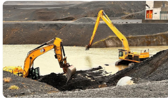
Dredging the drainage channel.
