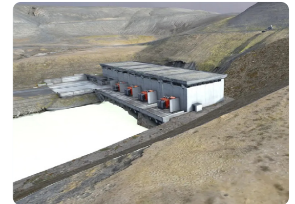
The station was originally designed for four turbines.
