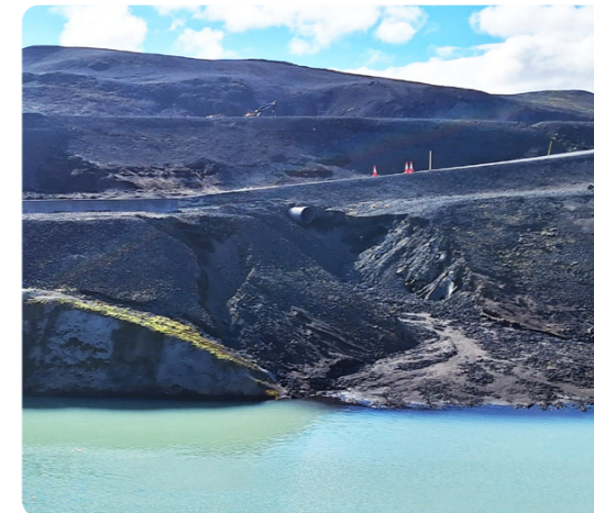
The crack branched and in places was clearly open.
