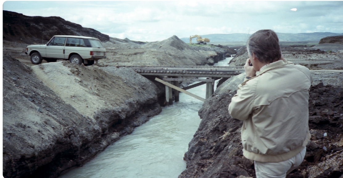
Construction at Búrfell in 1976.
