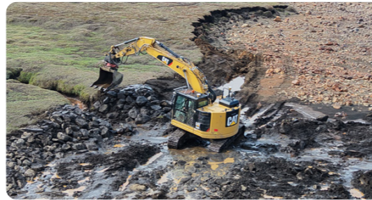
Bank protection work at Kringilsárrani, within the Háslón reservoir area. The bank protection is intended to protect a sensitive area by the reservoir.
