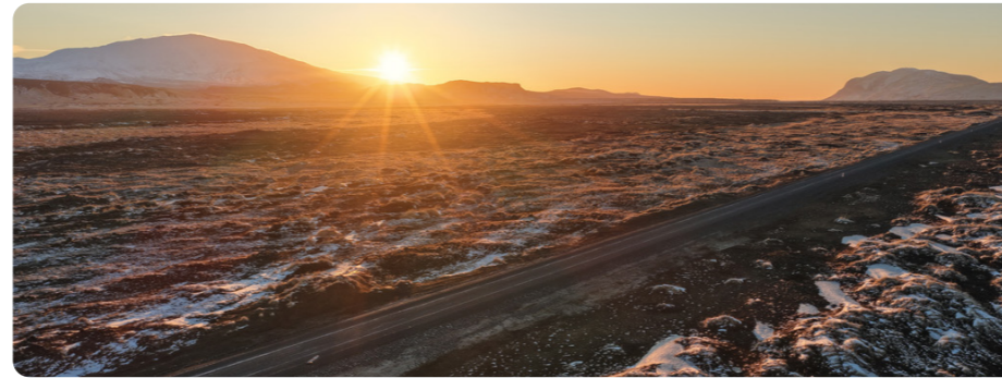
Work has been under way on improvements to Landvegur in connection with the Vaðalda project.
