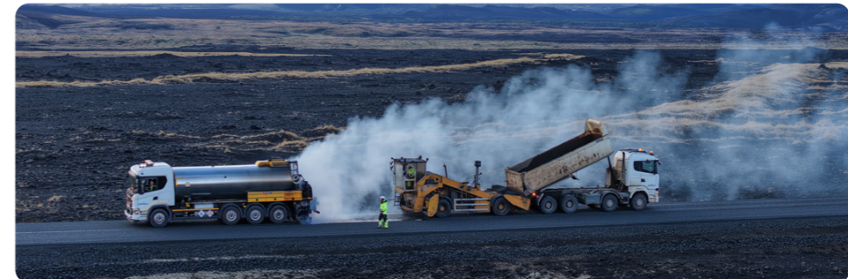
Landvegur road has been reinforced to enable the transport of the wind turbines.
